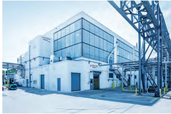
Siegfried USA, LLC 33 Industrial Park Road Pennsville, NJ 08070 USA
